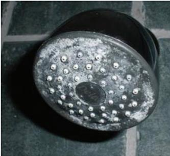
On the left is a photo of the showerhead in the left hand cubicle of the women's locker room on October 1st, 2009. The scale on the showerhead was hard and encrusted and could only be removed by using an acid cleaner.
